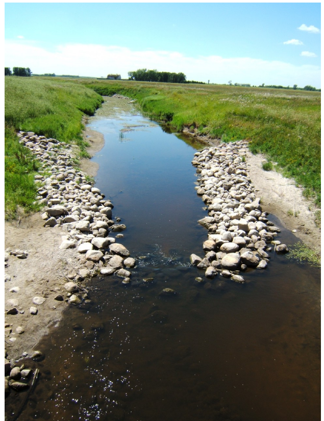
Gully 6 Erosion Control Site – August, 2005
